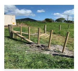
Good example of a corner setup. It can make more sense to minimise the number of corners on a strain length - strain the fence on a suitable corner, then fit another stay in the new direction and tie on the next section.
