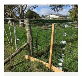
It is not a good idea to attach a new fence to an old one. When the strainer breaks, the new fence will fall over.
