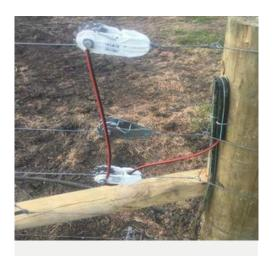
Terminal ties fitted correctly and all electric components fitted so cattle can't play and break. Wires clamped or crimped to achieve high quality connections.
