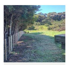
When possible, new fencing should be placed outside the drip line of the trees. In this example, the old fence can be seen against the trees and the new fence has been moved out to minimise damage to the bush line and some trimming has also taken place.
