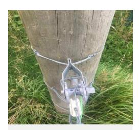
This is an example of permanent strainers not tied in correctly. A terminal tie should be used then tied through the end of the strainer with a minimum of five twists around the wire or crimped to achieve high quality connections.
